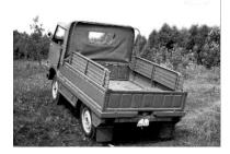
Lesser-known models from ŠKODA AUTO's 125-year history: Type 998 'Agromobil' from 1962 The ŠKODA Type 998 'Agromobil' featured a 1.98 x 1.59-metre platform body with a 1.24-metre-high tarpaulin that spanned the 3.9 m<sub>3</sub> loading space. Despite the positive test results, the compact all-wheeldrive vehicle, which was very agile off-road, never made it to series production.
